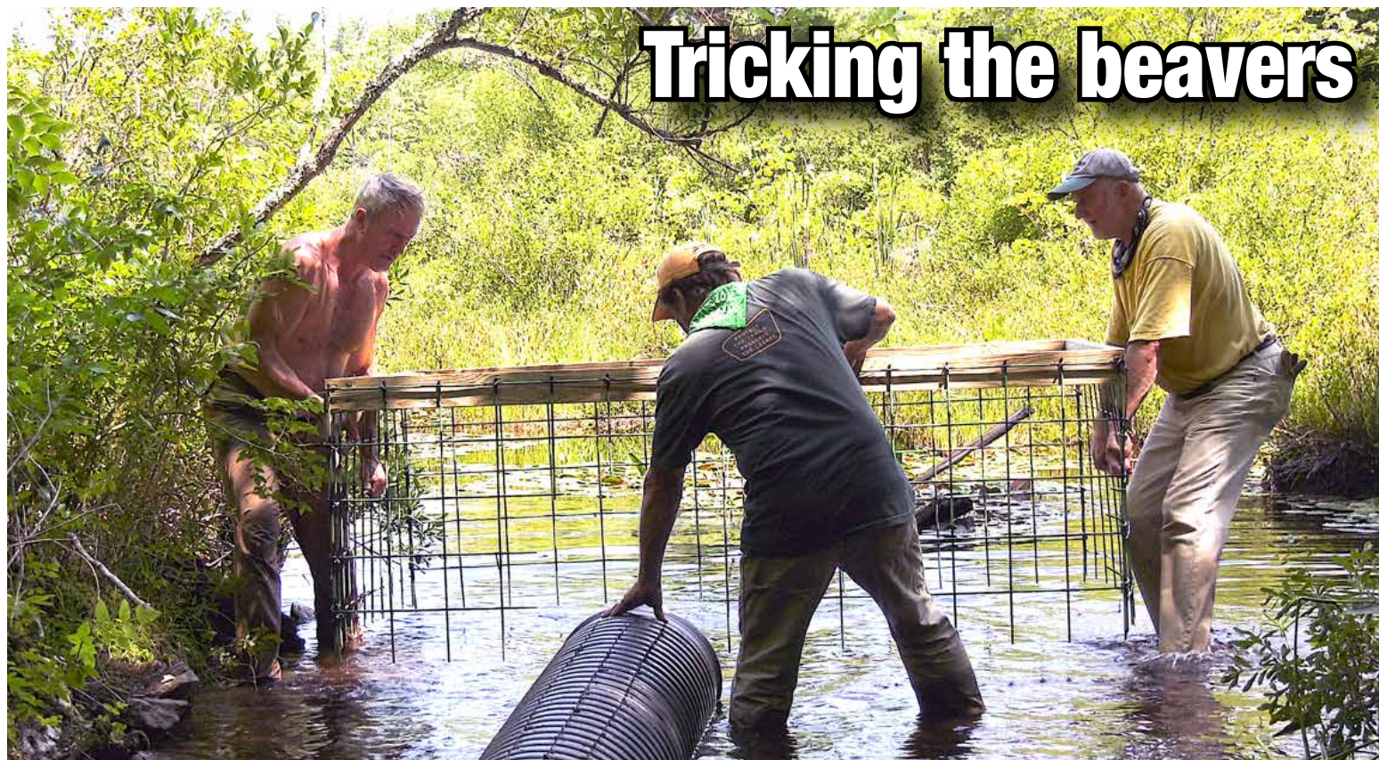
A filter box part of a "Beaver Deceiver" being installed on Deering Pond by Skip Lisle, Steve Mallon and Kevin McKeon to control beaver damage at a Mousam Way Land Trust property. COURTESY PHOTO
