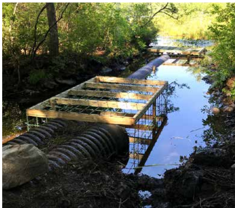
Culvert Fence (Culvert Box): protects culverts from beaver damming.
