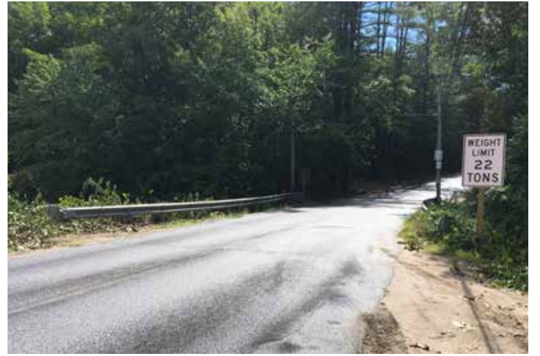
View of Emery Mills Bridge to be replaced, with new 22 Ton Limit.
