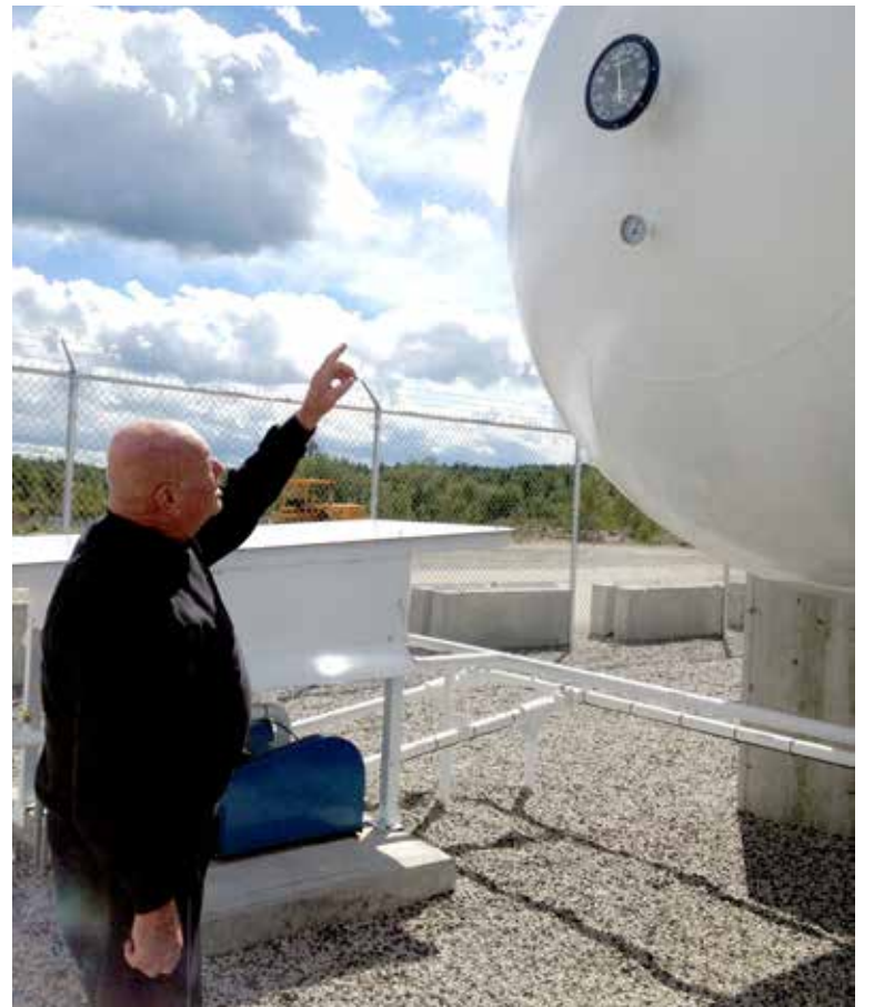
Frank Carroll points to the pressure and fuel level gauges on his propane storage tank located at F.R. Carroll. COURTESY PHOTO
