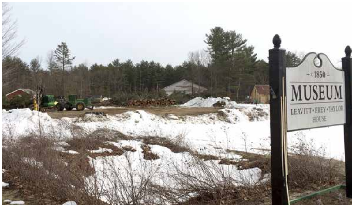
Softwood trees surrounding the Waterboro Central Fire Station property have been cut down as a matter of safety and aesthetics. PHOTO BY KERRY DEANGELIS
