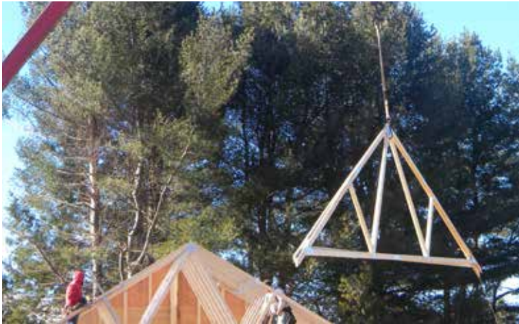
Roof rafters are carefully put in place during the construction of the annex to Henry Hall at the Brothers of Christian Instruction in Alfred.
